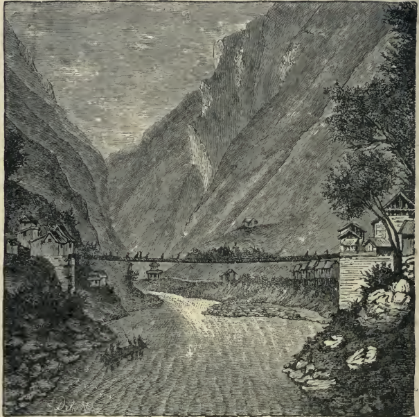
Iron Suspension Bridge at Lowatong. (From Garnier.)
