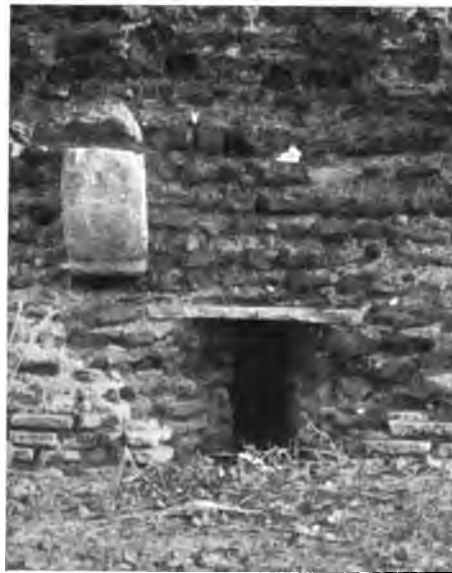
Fig. 140.—Rome. Villa called "Sette Bassi." Double-splayed window (100–155).
