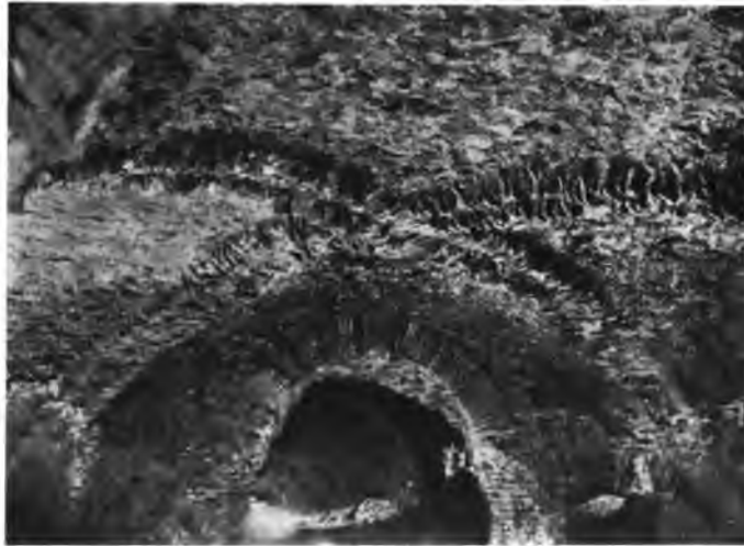
Fig. 362.—Rome. Villa called "Sette Bassi." Ribbed vaulting (IIInd Century).
