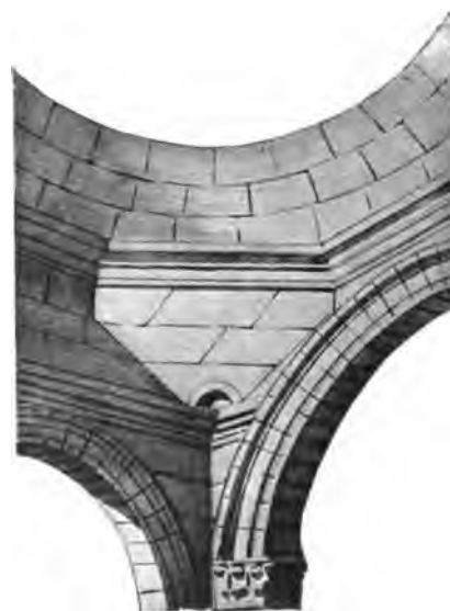
Fig. 275.—Lattakia. Angle raccord in four-faced arch (IIIrd Century).
