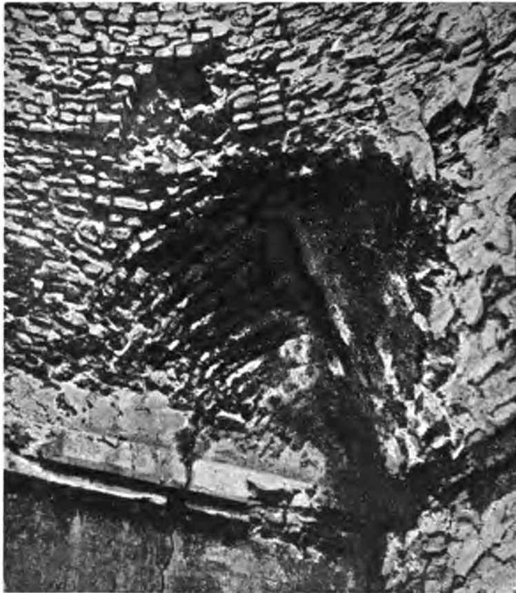
Fig. 276.—Firuz-Abad. Angle raccord in palace. (From Dieulafoy, " L'art antique de la Perse .")
