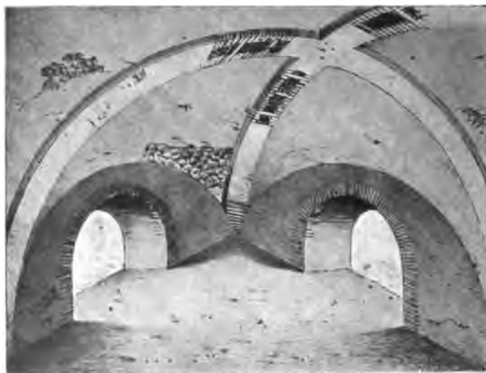
Fig. 361.—Rome. Villa called "Sette Bassi." Ribbed vaulting (IIInd Century).
